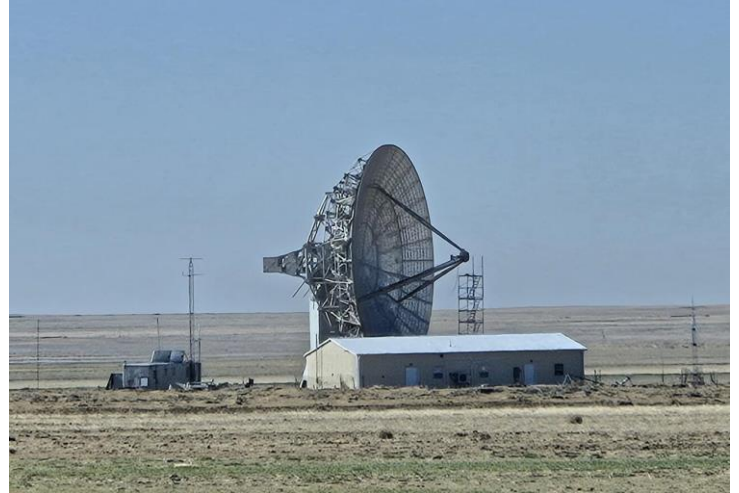
Figure 1: DSES 60' Dish and New Control Building
