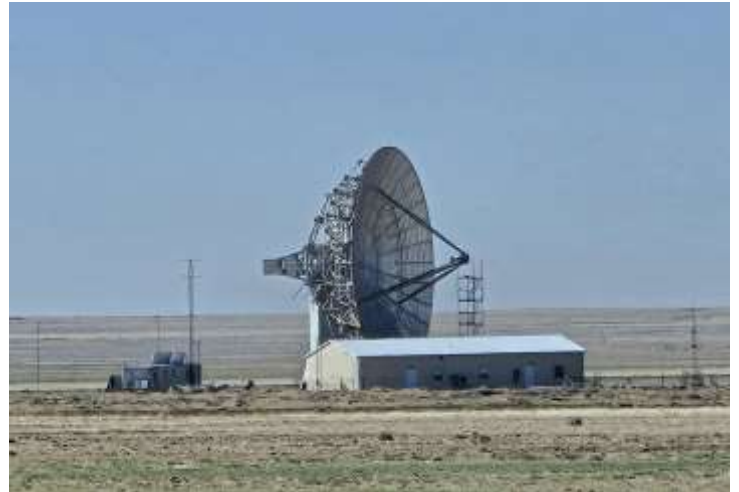
Figure 1: DSES 60' Dish and New Control Building
