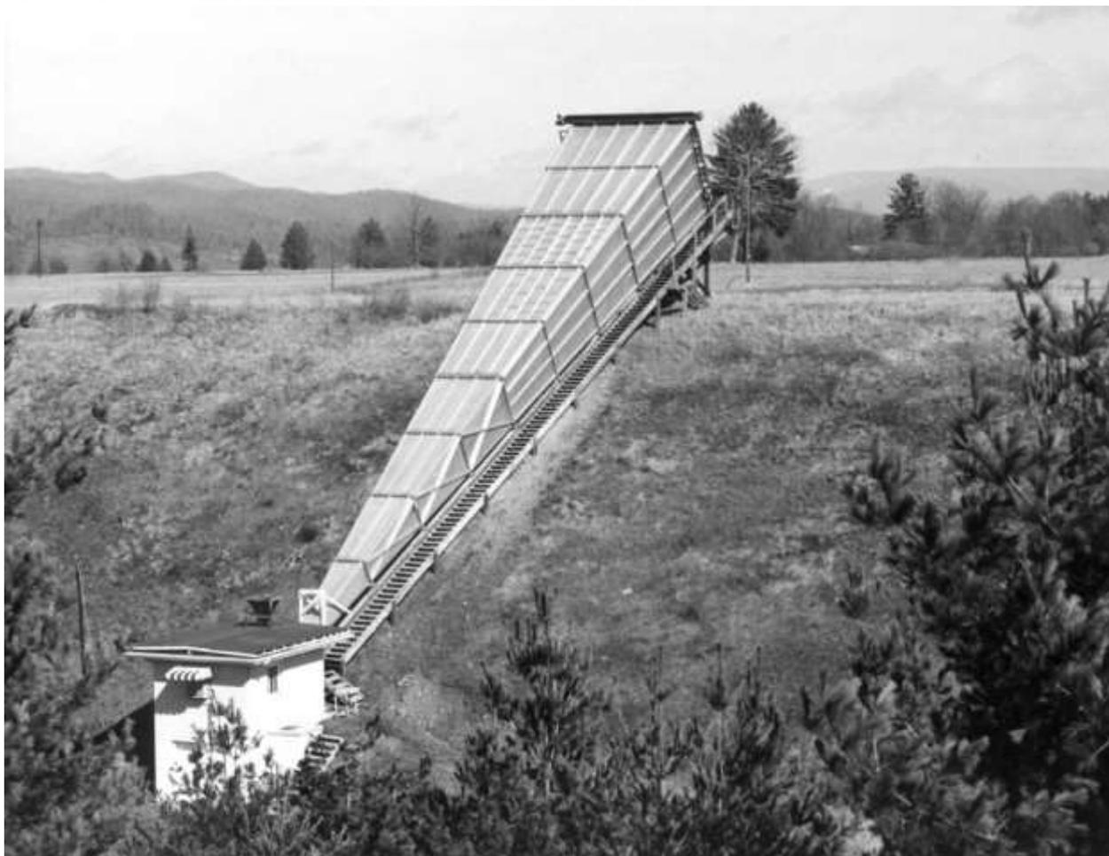
The 13 foot x 17.5 foot aperture end of the 120-foot long Calibration Horn Antenna, otherwise known as the “Little Big Horn,” at Green Bank. It was built in 1959 to observe the sky’s strongest non-solar radio source, Casseopeia A, and measure its total power output at a frequency of 1.4 GHz (L-band, 20cm wavelength). It was also used to map Cas A’s spectrum and take absolute temperature measurements of the background sky. [ circa 1967 NRAO/AUI/NSF text/image]
