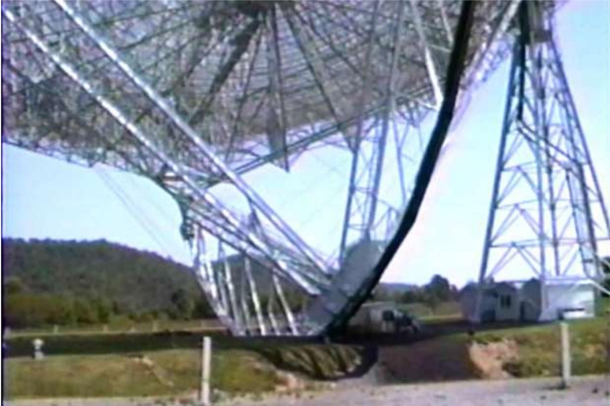
Drive gear and counterweight below the 300ft transit dish in June 1988. November 15<sup>th</sup>, 1988, the dish collapsed due to a gusset plate stress fracture which had been cracking slowly for a long time. The dish was put up as a temporary antenna due to delays in the completion of the 140ft dish twenty-five years before. The 300ft telescope was built in 1962.
