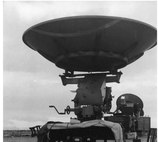
465 mc apparatus (10 foot radar mirror)
