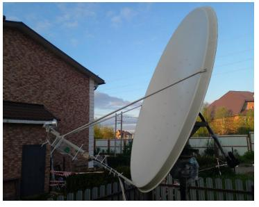
Figure 2. Methanol maser telescope 6.7 GHz (2023).
