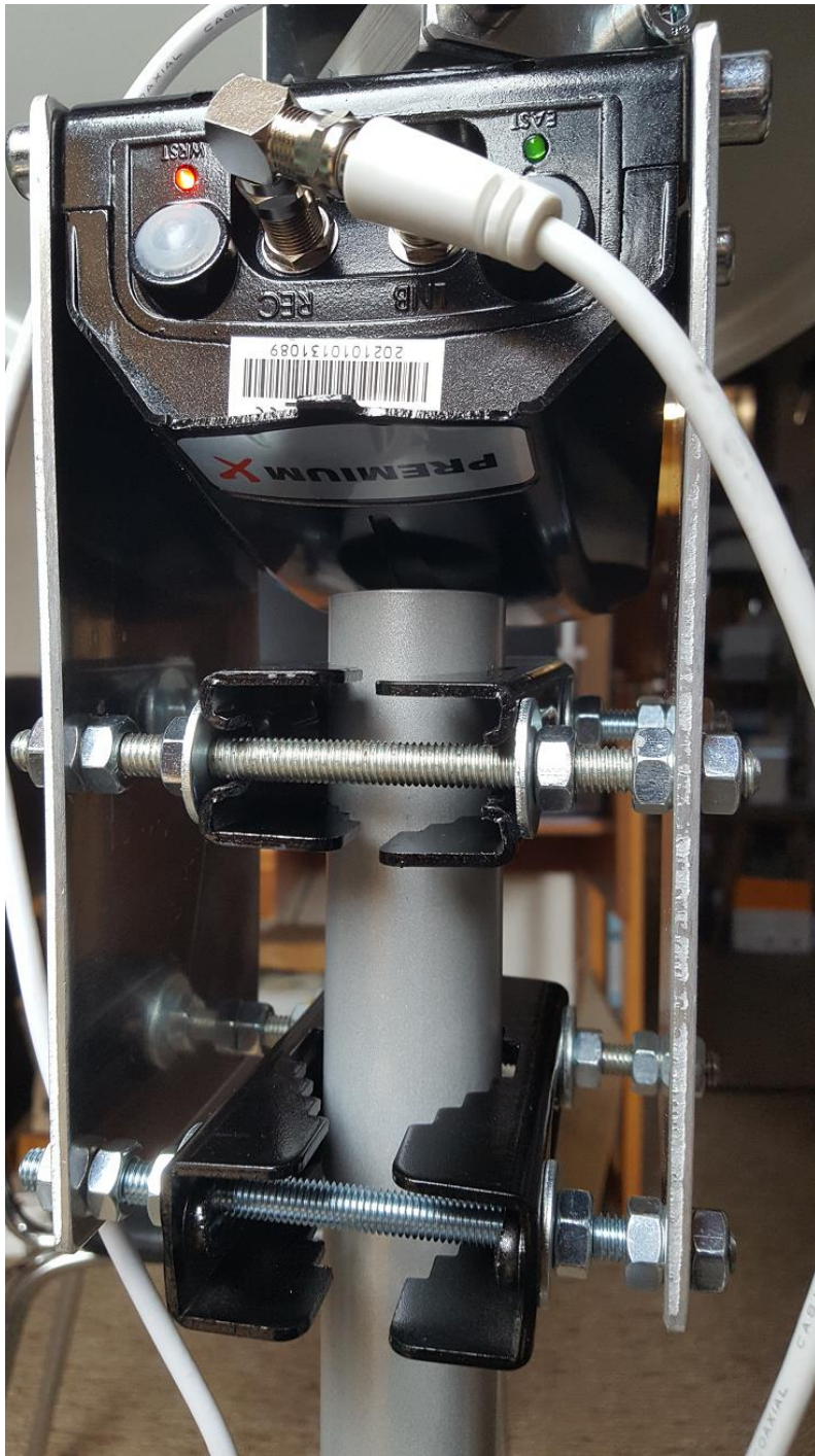
Figure 2 ~ Detail view of the azimuth rotor fixation on top of the tripod pole.
