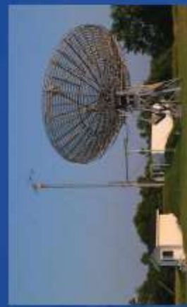
SARA members have been privileged to use this forty foot diameter drift-scan hydrogen line radio telescope every year at their annual meeting in Green Bank.
