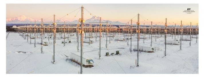
Figure 8 ~ View from a drone at about 13.8 m (50 ft) altitude of the Ionospheric Research Instrument – crossed-dipole antennas and transmitter enclosures – as the Sun was setting at the HAARP facility. Mount Drum, part of the Wrangell Mountains, is in the middle far background. This image was taken near the same location as the opening image in this article but at a lower altitude. Image courtesy of UAF-GI.
