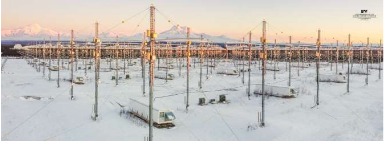
Figure 8 ~ View from a drone at about 13.8 m (50 ft) altitude of the Ionospheric Research Instrument – crossed-dipole antennas and transmitter enclosures – as the Sun was setting at the HAARP facility. Mount Drum, part of the Wrangell Mountains, is in the middle far background. This image was taken near the same location as the opening image in this article but at a lower altitude. Image courtesy of UAF-GI.
