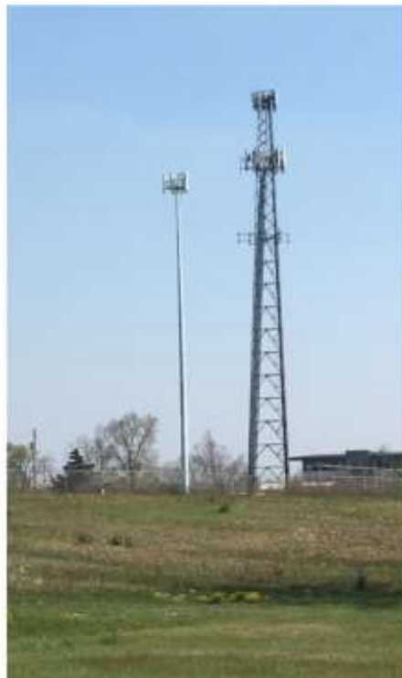
Figure 5: Cell Towers Producing LNA Overload
