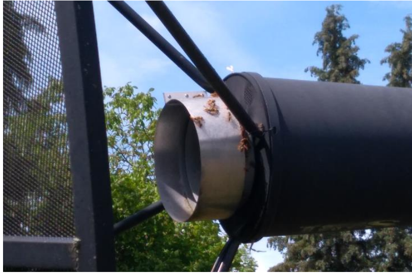
Figure 2: Not a good idea to dismantle at that moment
