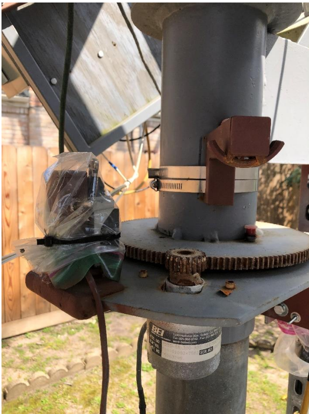
Figure 3: Azimuth Motor Drive
