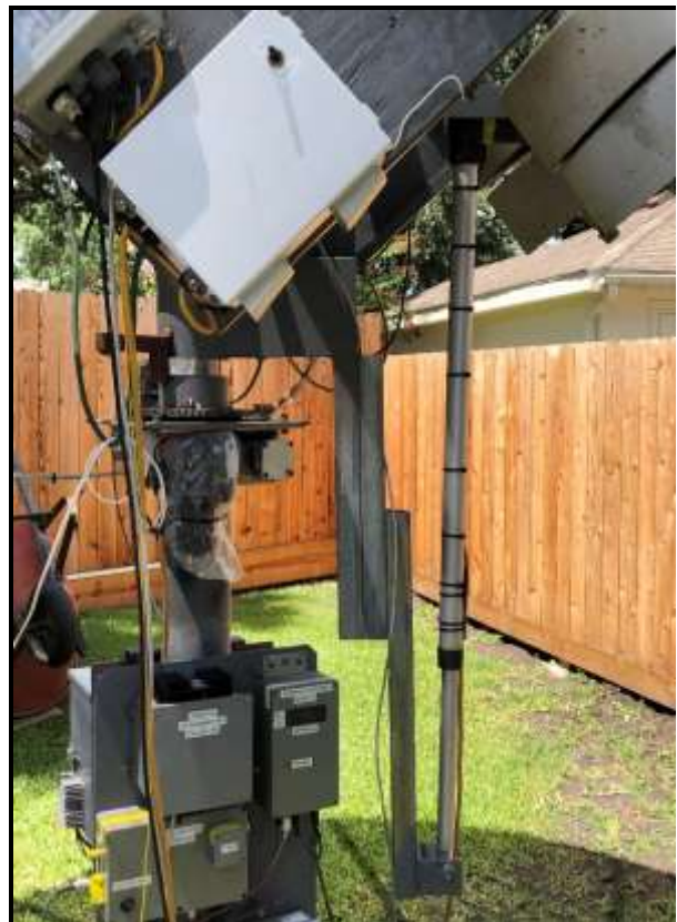
Figure 4: Altitude Motor Drive
