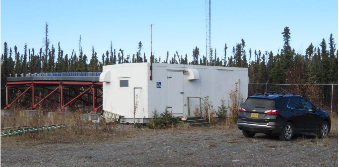
Figure 3 ~ MUIR equipment enclosure and associated radar antenna array (left-background). All electronics for the Callisto-LWA Antenna installation were placed in the enclosure at the end of September. A protected coaxial cable entrance facility was installed on the back of the enclosure (not visible in this picture). This picture was taken the day before the weather station and lightning sensor was installed on the enclosure. Image © 2021 W. Reeve
