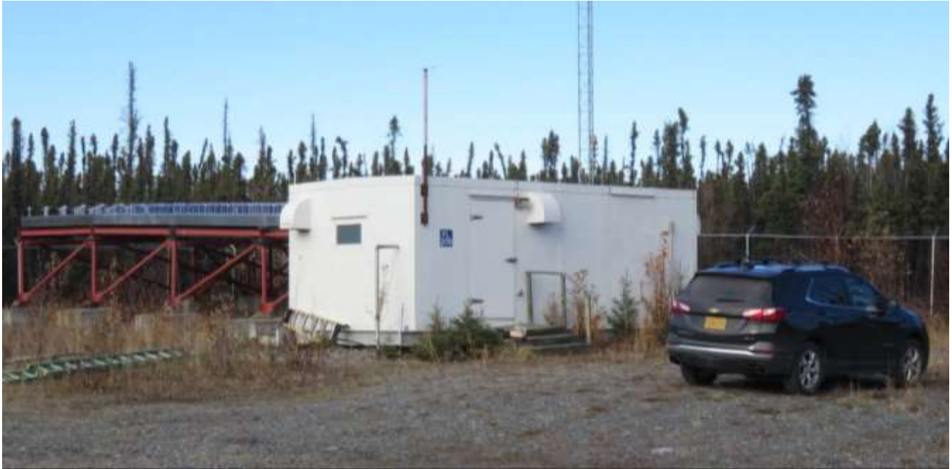
Figure 3 ~ MUIR equipment enclosure and associated radar antenna array (left-background). All electronics for the Callisto-LWA Antenna installation were placed in the enclosure at the end of September. A protected coaxial cable entrance facility was installed on the back of the enclosure (not visible in this picture). This picture was taken the day before the weather station and lightning sensor was installed on the enclosure. Image © 2021 W. Reeve
